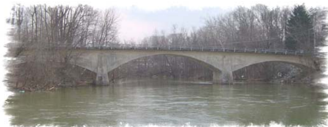
Panhandle Road Bridge over Olentangy River (the Stone Mill Bridge)
